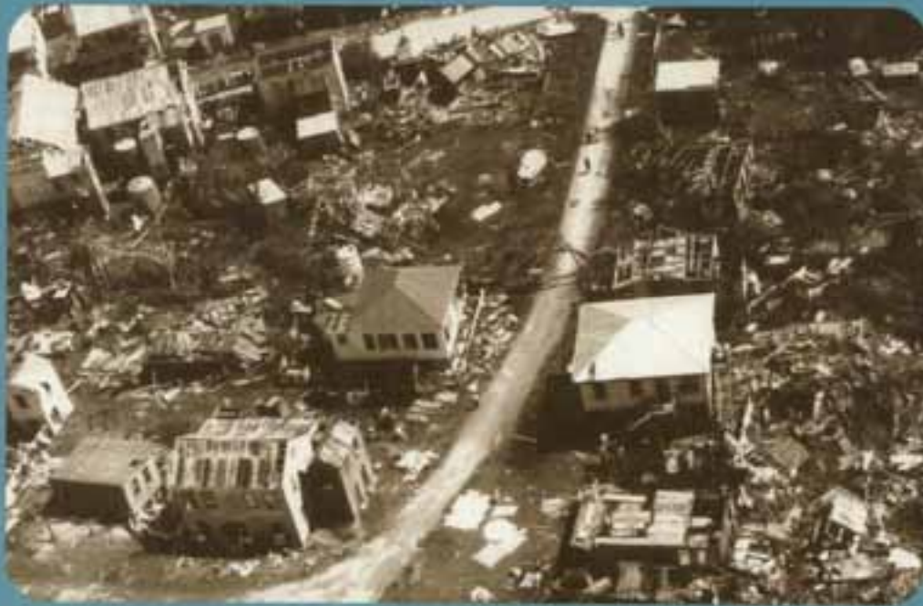
Aerial view of the devastation caused by Hurricane Hattie, October 1961
